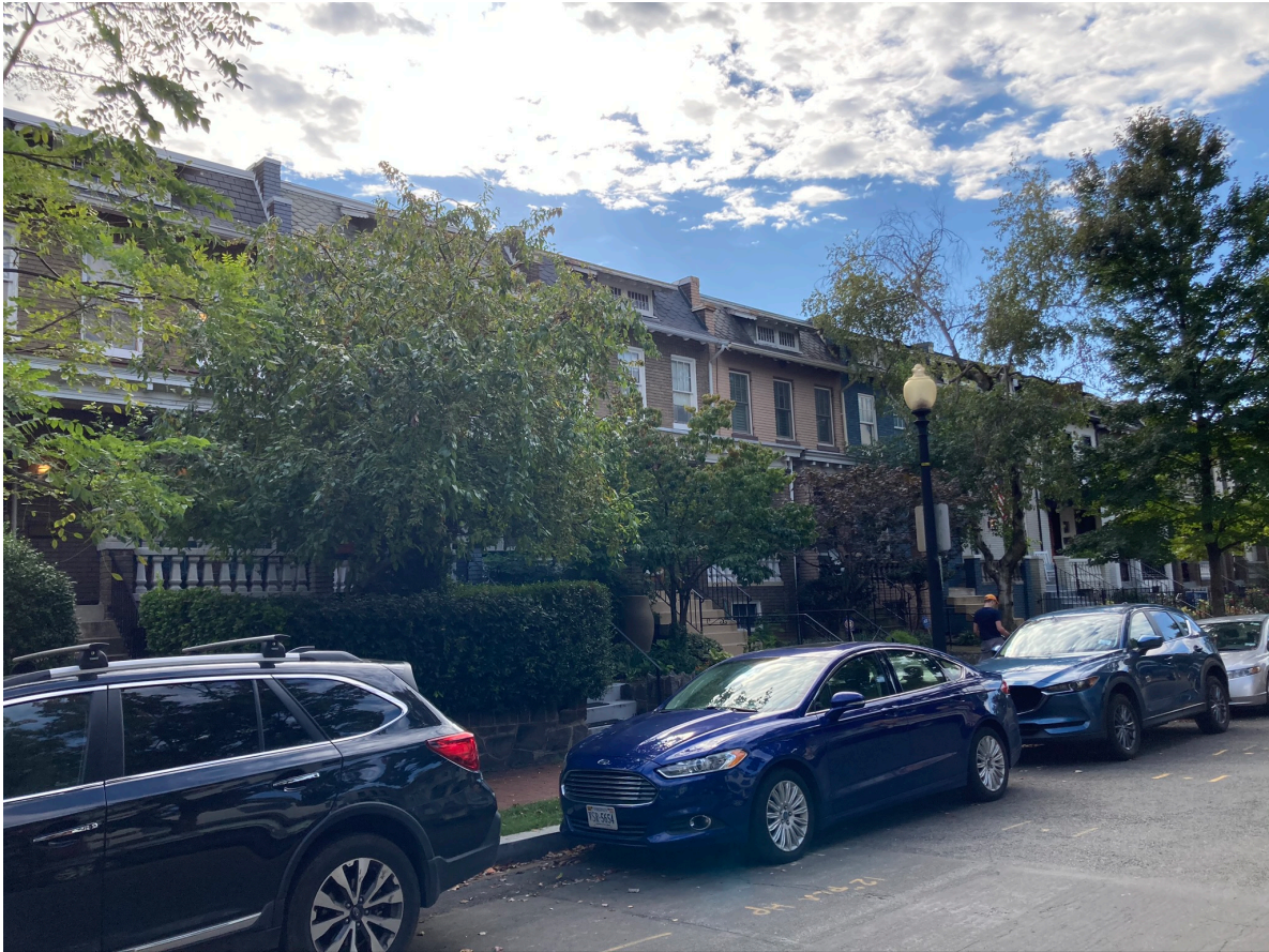
NORTH VIEW, 10 TH STREET SE
