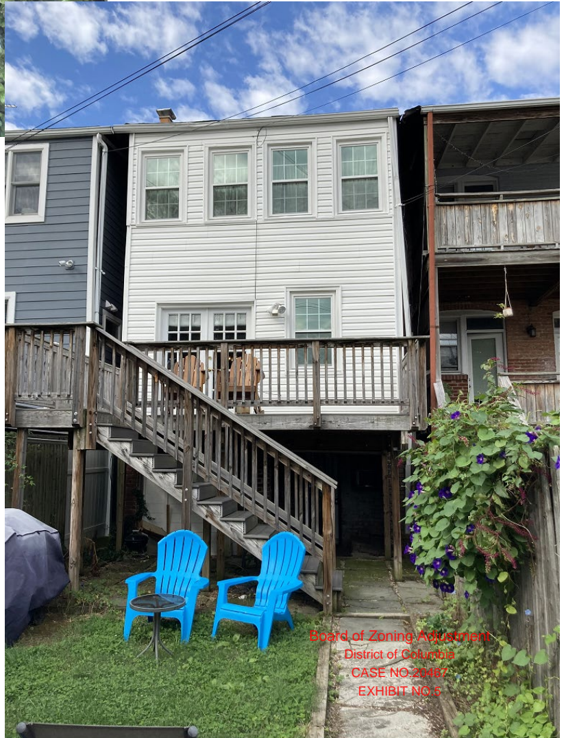
EXISTING REAR FACADE
