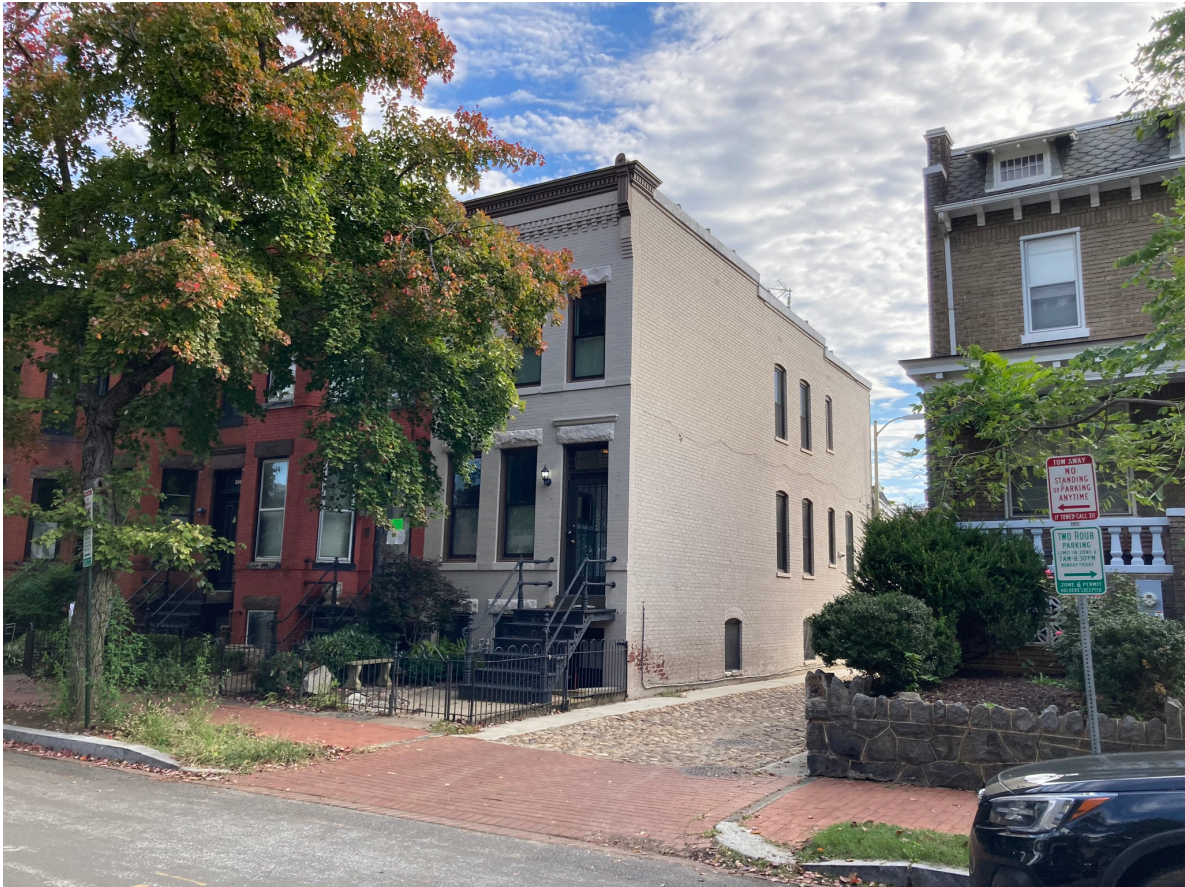
SOUTH VIEW, 10 TH STREET SE
