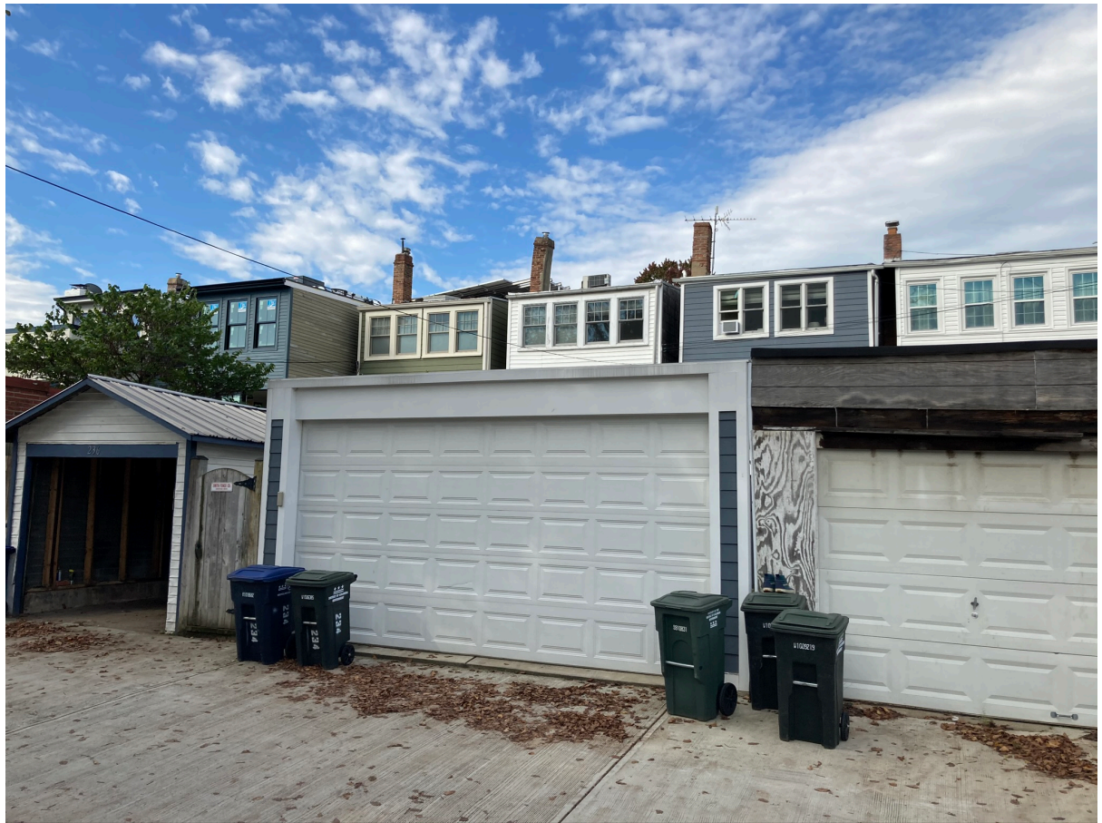
ALLEY NORTH VIEW
